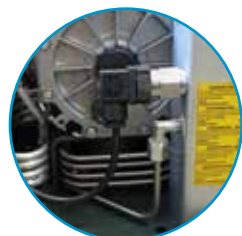
Pressure switch for automatic stop
