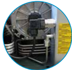
Pressure switch for automatic stop
